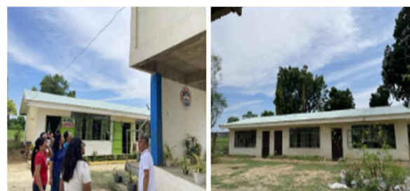
Fig. 10. Left: Pilig Alto Elementary School's Principal and Teachers providing information on the level of the highest recorded flood height at 3.5 meters just right above the top of beam of the school stage, right: unused building of the school due to extent of damage caused by the previous typhoon
