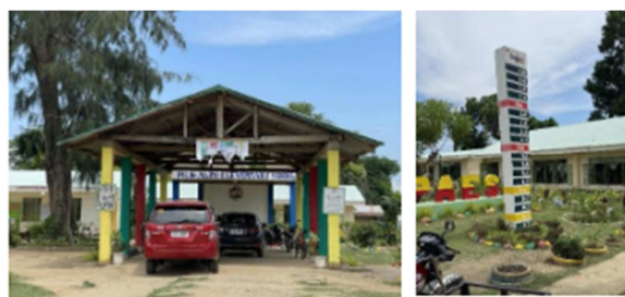
Fig. 9. Left: Pilig Alto Elementary School Multi-Purpose Hall, right: presence of flood ground marker as early warning advisory of the school
