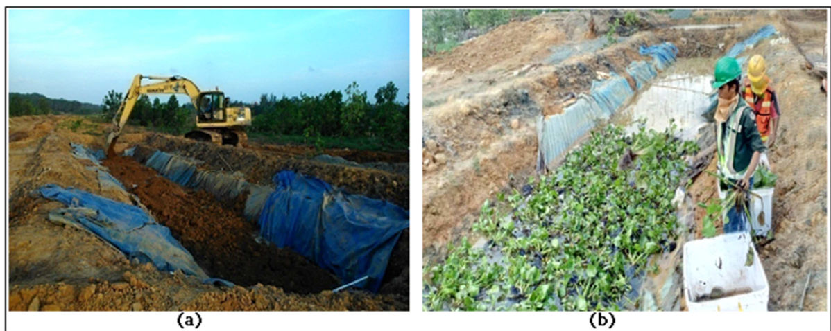
Fig. 2. (a) Bokashi allotment in CW, (b) CW with Wh and Cwc plants.
