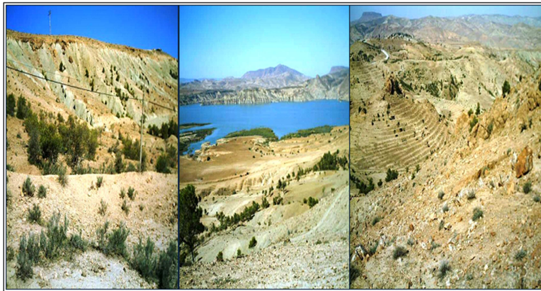
Fig. 1. Sidi M'hamed Benaouda Dam and landscape in the study area.
