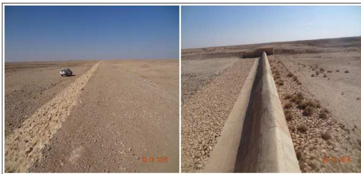
Fig. 7. Submersible dam that built on the wade Hasoub cross-section.
