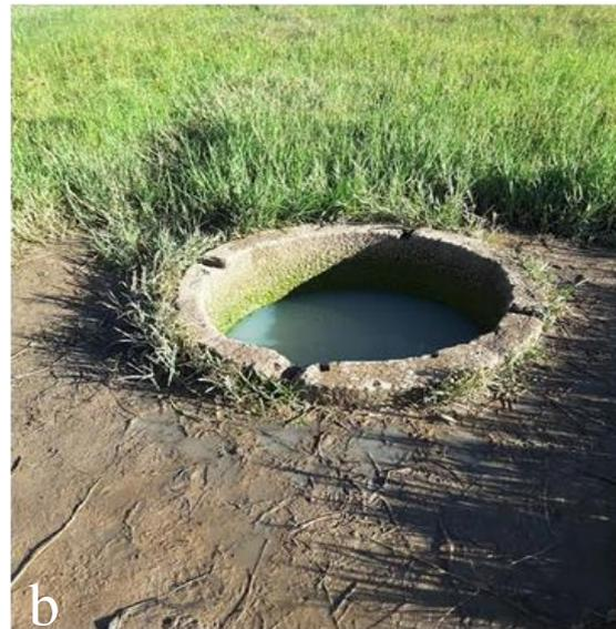
**Plate 1.** Type of covers and well condition observed from the study area: (a) fractured metal cover (b) uncovered wells with poor well-head elevation, lack fence and possess unhygienic surrounding.
