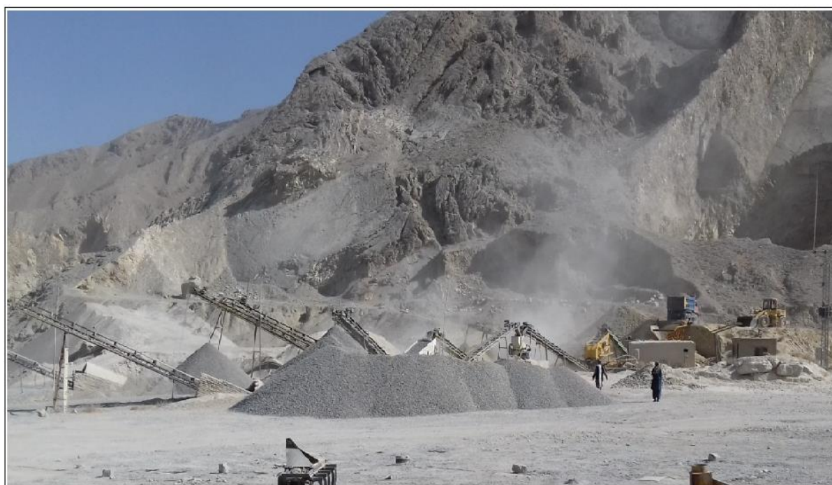
Fig. 1. Abbaseen stone crushing plant at Kuchlak Quetta.
