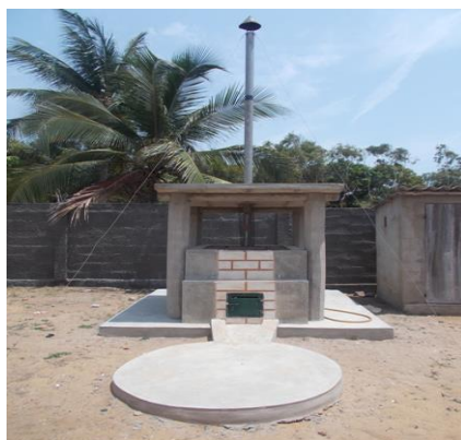
Figure 4. Non-electric artisanal incinerator.
