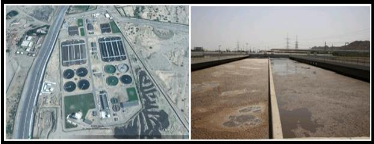
Fig. 1. Haddah Sewer Treatment Plant (HSTP) in working condition.
