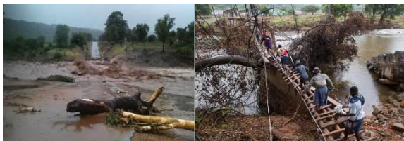
Plate 4. Damaged Chimanimani tarred road and a temporary crossing structure at Nyahode River.
