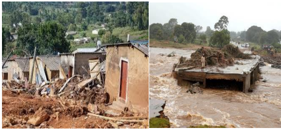
Plate 3. Chimanimani- Ngangu resident house and Nyahode Bridge swept by Cyclone Idai floods.
