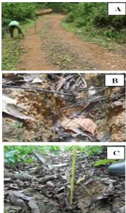
Fig. 4. Gap of vegetation created by wheels. A, AAC 2010 at 20 % of slope; B, AAC 2009 at 15 % of slope (drain formed after 2 years); C, AAC 2009 at 15 % of slope (see the depth of the drain).
