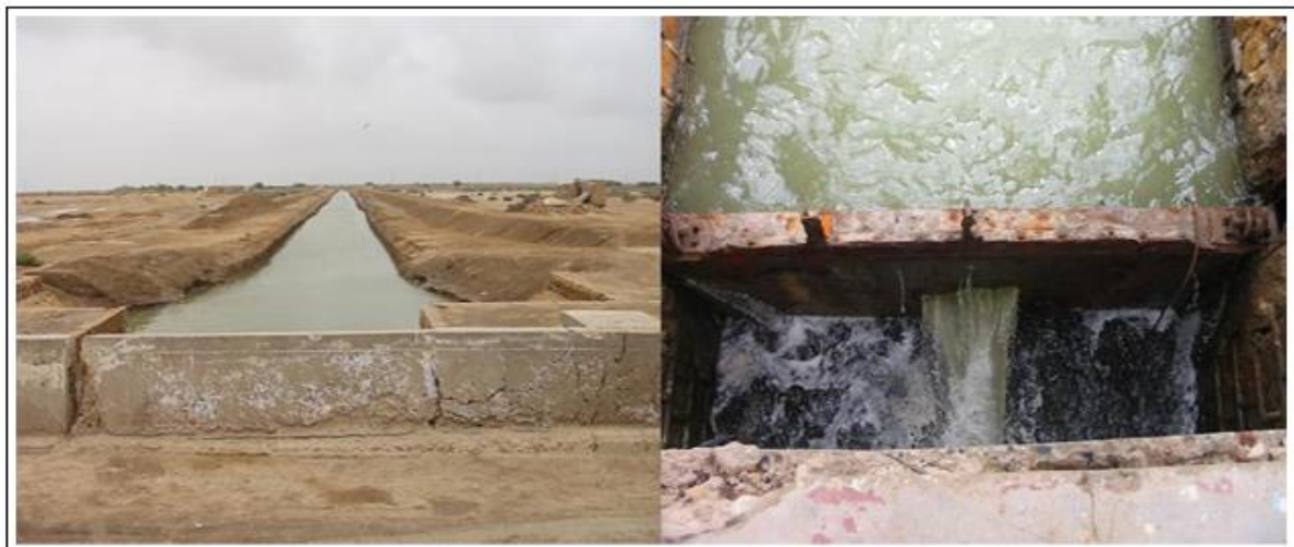
Fig. 4. Sea water intrusion through the network of canals constructed for the discharge of saline ground water to the sea.
