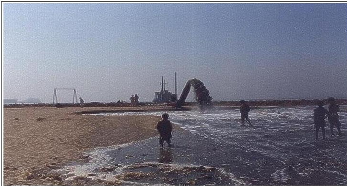
Fig. 9. Dredging of sand from low water line.
