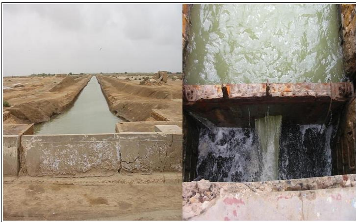
Fig. 12. One of the drainage canals in the Indus deltaic area of Ketu Bunder where the sea water is entering into the irrigation land through the faulty gate. (Muzaffar et al , 2017).
