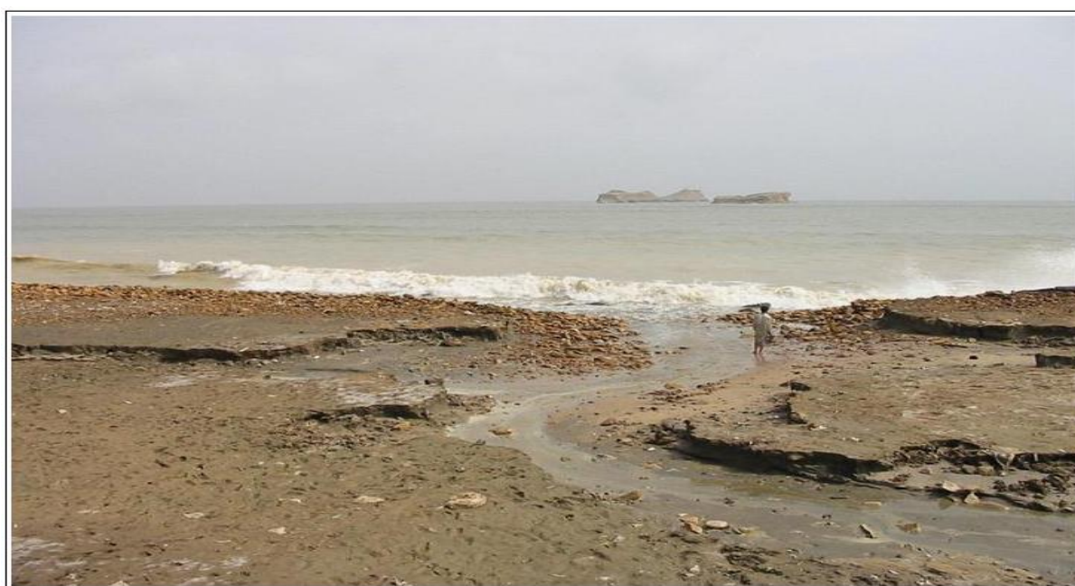
Fig. 11. Destruction and incision of Marine Drive, Clifton Beach Karachi due to high wave action.
