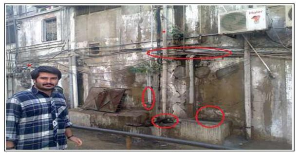
Fig. 7. Shows drinking water pipes association with sewage line (Block 6).
