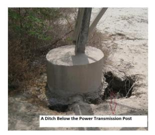
Fig. 4. Development of a ditch.
