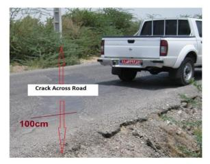
**Fig. 3.** Passing of crack across road in Chelo Gavmishi village.
