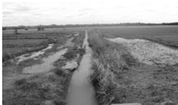
Picture 2. Showing broken laterals.
