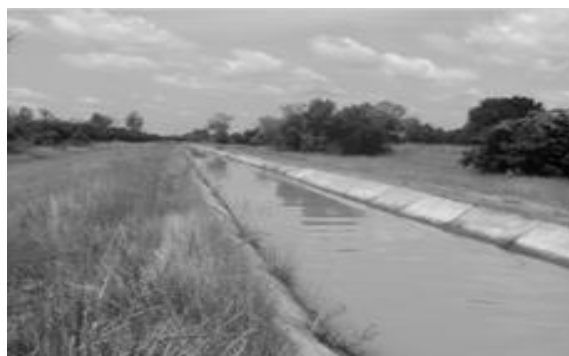
Picture 3. Showing the rehabilitated main canal.
