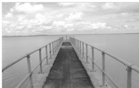
Picture 1. Showing Tono reservoir.
