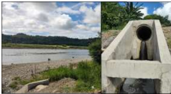
Fig. 12. Drainage directly discharging wastewater beside Station 6
